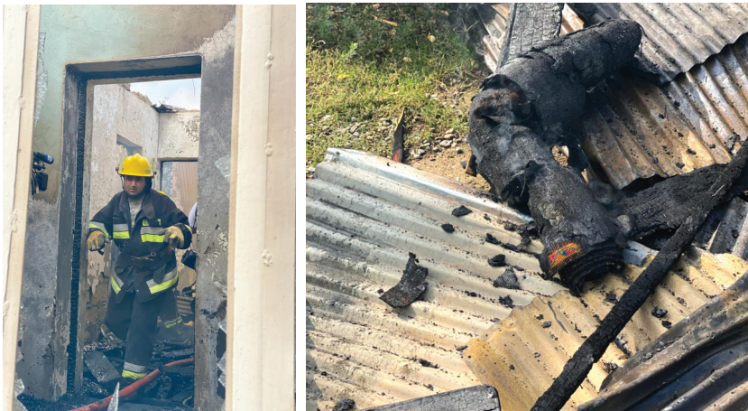
A house in Aghdam district (Azerbaijan) completely destroyed by fire.
