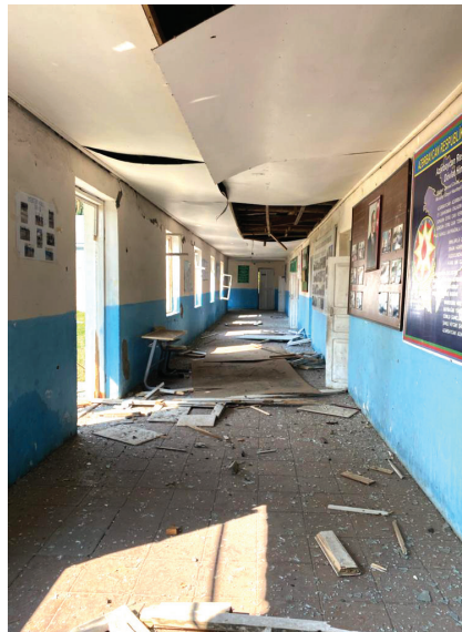
Shelling of school building in Eskipara village of Terter district, Azerbaijan
